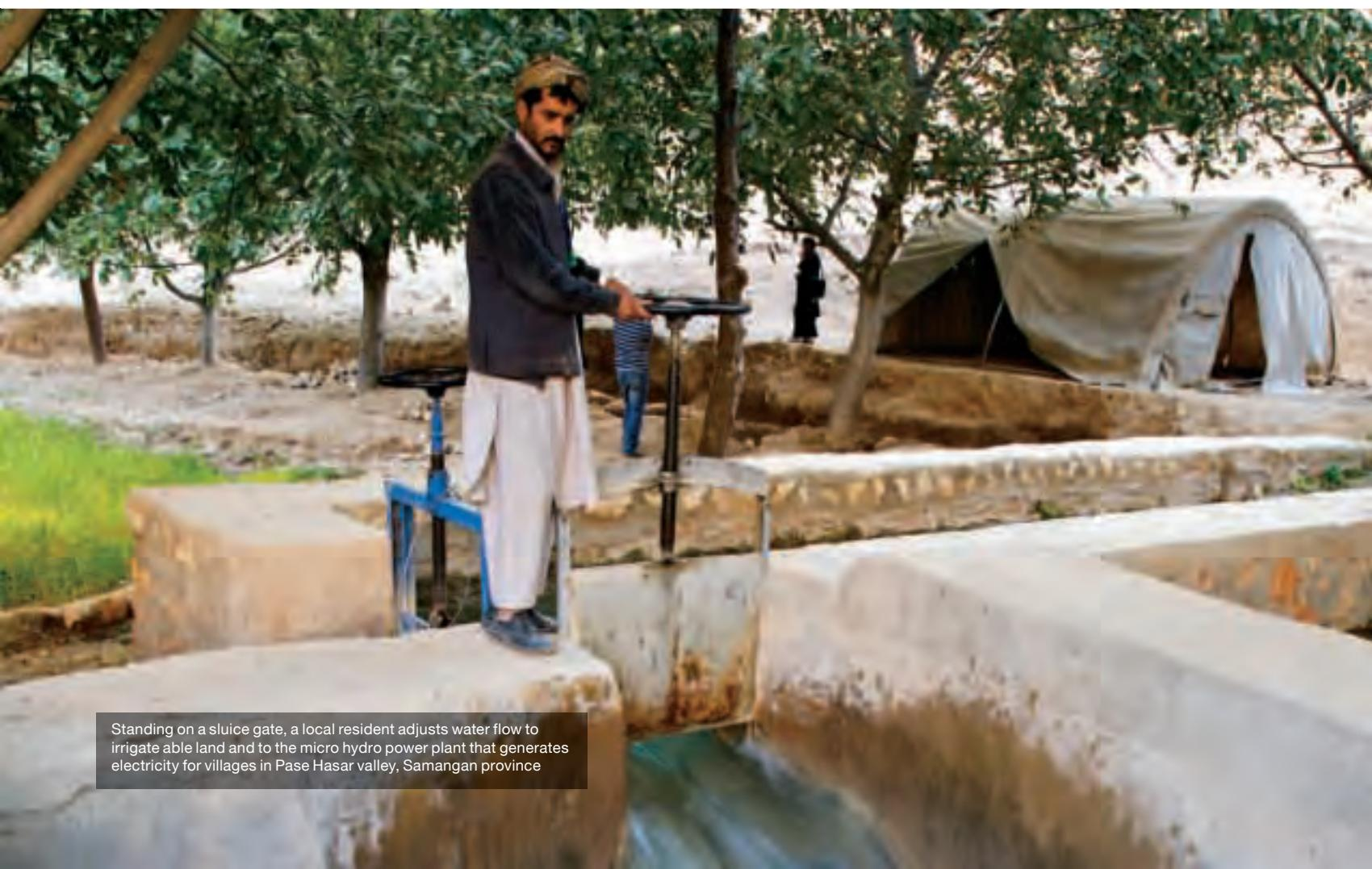
Standing on a sluice gate, a local resident adjusts water flow to irrigate able land and to the micro hydro power plant that generates electricity for villages in Pase Hasar valley, Samangan province
