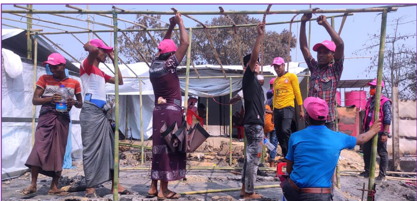
Community group members helping to reconstruct the damaged shelters
