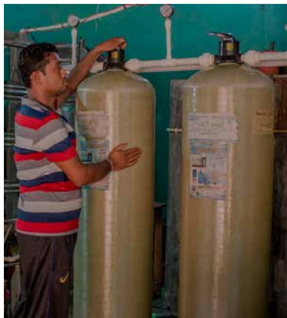
Reverse osmosis technology-based water treatment plant
